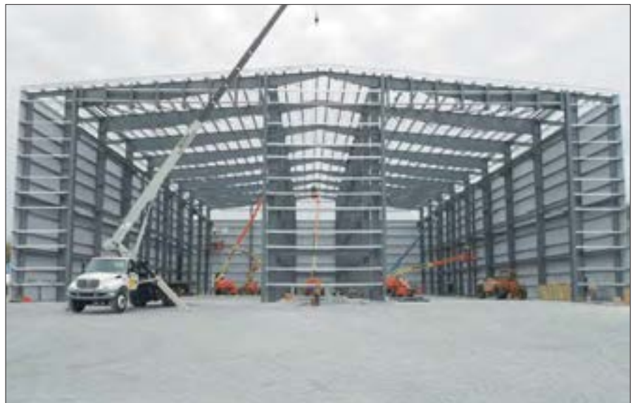
Building No. 5, shown on the article's opening page, seen here in frame. Maine Coast Construction Co., based in Camden, erected, renovated, or supplied the materials packages for all the yard's buildings—and did so on an exceedingly tight timeline.
