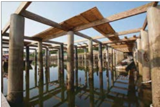
Left —Front Street “inherited” an unfinished and thus languishing marina project. Most of its pilings had to be replaced. Right —One of the yard’s first priorities was to build a substantial pier for its 165-ton (150-mt) Travelift, with associated finger piers
