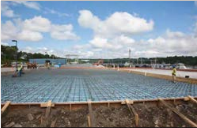
The concrete slab for what is currently Front Street's biggest building, called "No. 5," turned out to be, in the summer of 2011, the largest pour in the entire state since 2007—or just prior to the Great Recession. Designed to handle 300-ton (272-mt) loads, the slab required 1,336 cubic yards (1,021m 3 ) of concrete, reinforced by 175,000 lbs (79,379 kg) of rebar.
