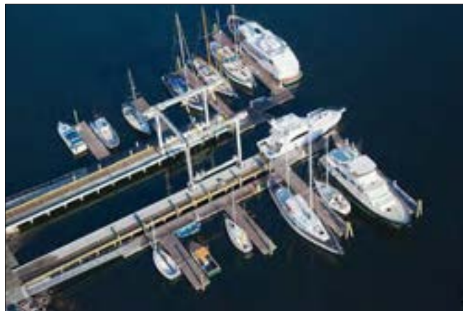
Left —Front Street “inherited” an unfinished and thus languishing marina project. Most of its pilings had to be replaced. Right —One of the yard’s first priorities was to build a substantial pier for its 165-ton (150-mt) Travelift, with associated finger piers
