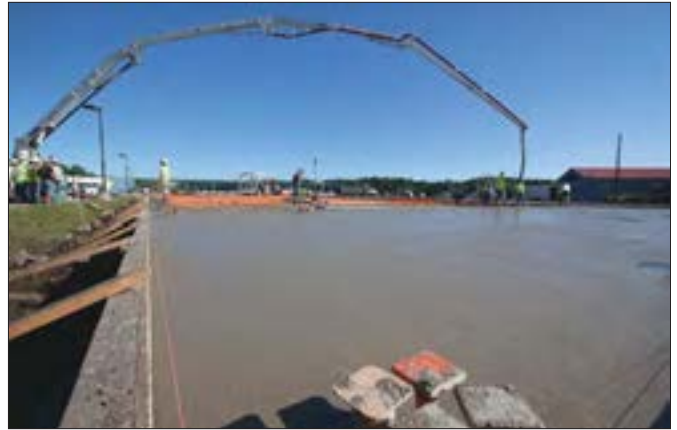
The concrete slab for what is currently Front Street's biggest building, called "No. 5," turned out to be, in the summer of 2011, the largest pour in the entire state since 2007—or just prior to the Great Recession. Designed to handle 300-ton (272-mt) loads, the slab required 1,336 cubic yards (1,021m 3 ) of concrete, reinforced by 175,000 lbs (79,379 kg) of rebar.
